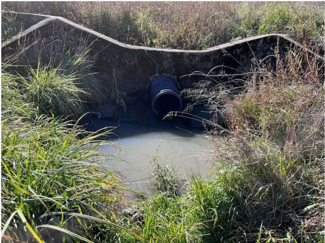
Stream IT 002 (Intermittent), facing upstream on October 27, 2022.
